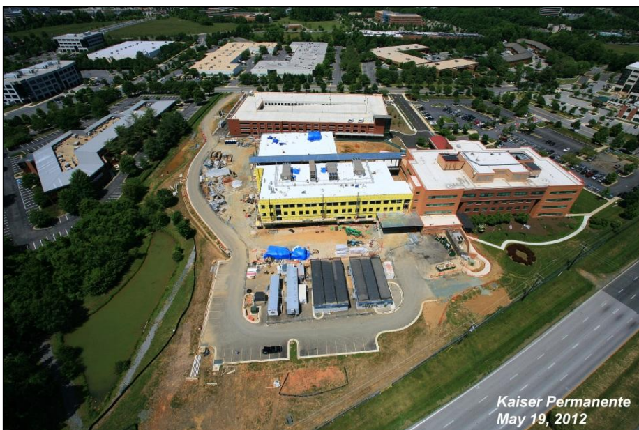
Figure 1 - The stormwater management pond protection can be seen in the lower left of the image. This area has been protected throughout construction and the pond will be completely restored upon completion of the project. Image courtesy of DPR Construction.
