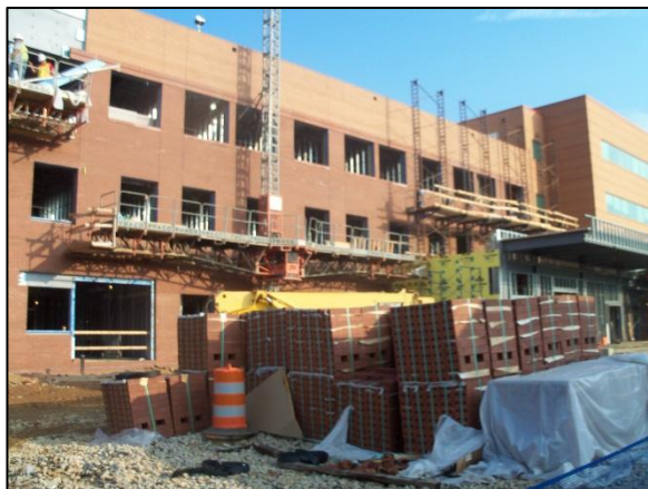
Figure 9 - Fraco Lifts which didn't allow work to be done underneath along with large amounts of brick taking up valuable laydown space for an extended period of time can be seen here. Personal photo taken by Chris Pozza.
