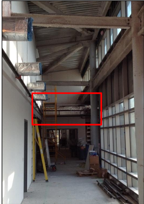
Figure 8 - View of corridor space in Area B on the third floor looking south. Ductwork can be seen crossing this space running from Area B to Area C along with the clerestory window in the upper right of the image. Personal photograph taken by Chris Pozza.
